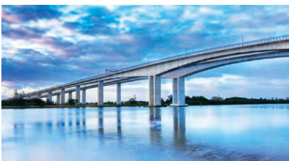
Monitor infrastructural deterioration in bridges
